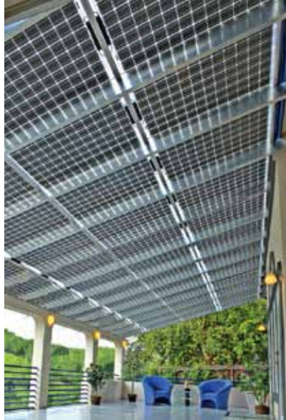
Patio Awning: Solar Living Design Lakewood, CO
